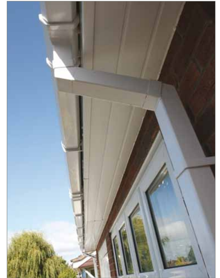
Square-line guttering shown in White
